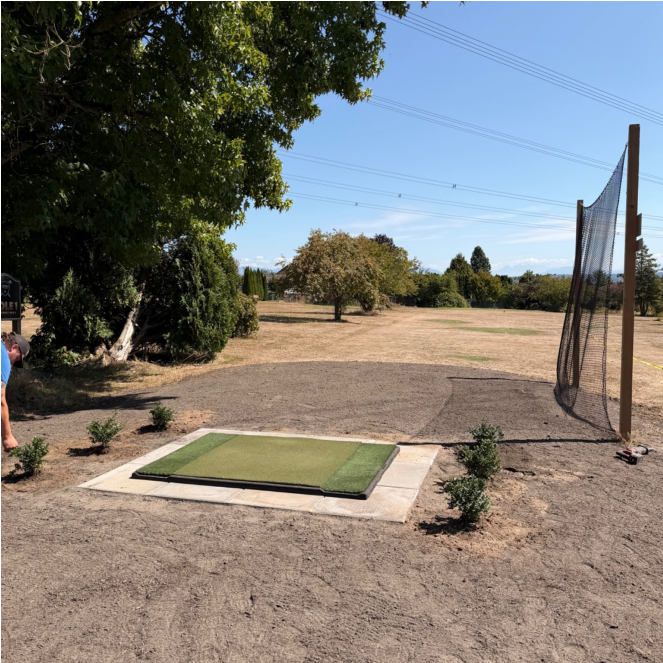
Tee Box #1: one of five tee boxes already rebuilt as part of the course revitalization project.
